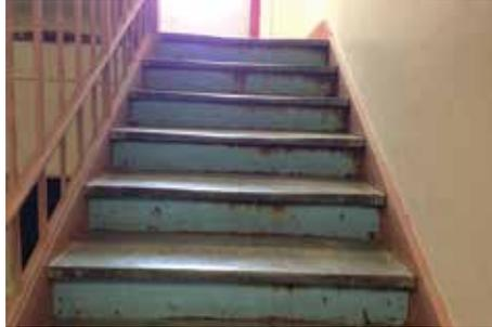
The stairway is rusted from water infiltration.
